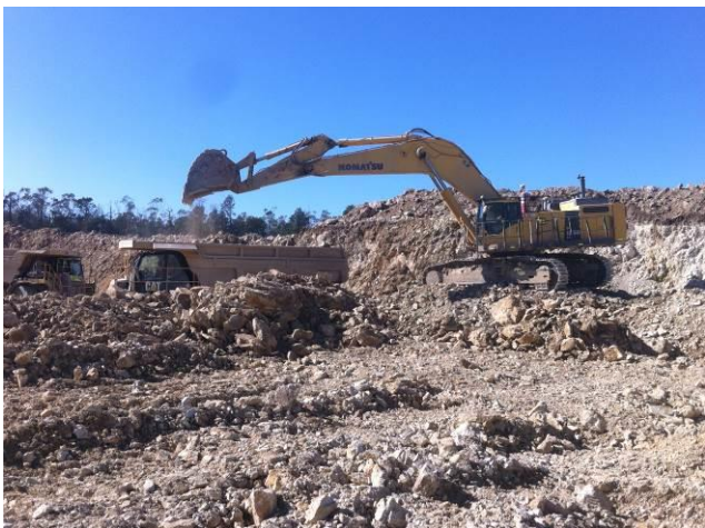
Figure 1. Pre Stripping at Pearse Open Pit
