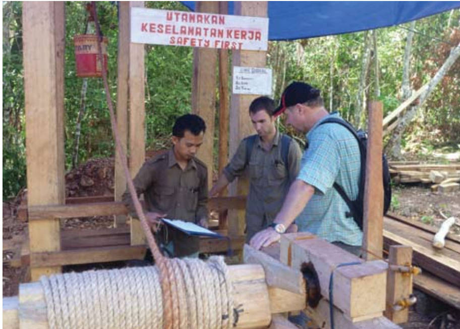
Shaft construction at Batu Hitam, Lakuwahi Prospect
