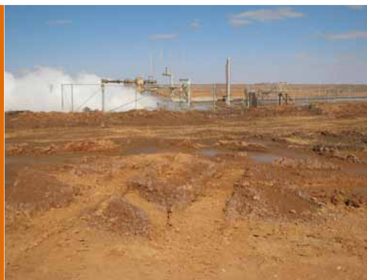
Habanero 3 well site during the incident
