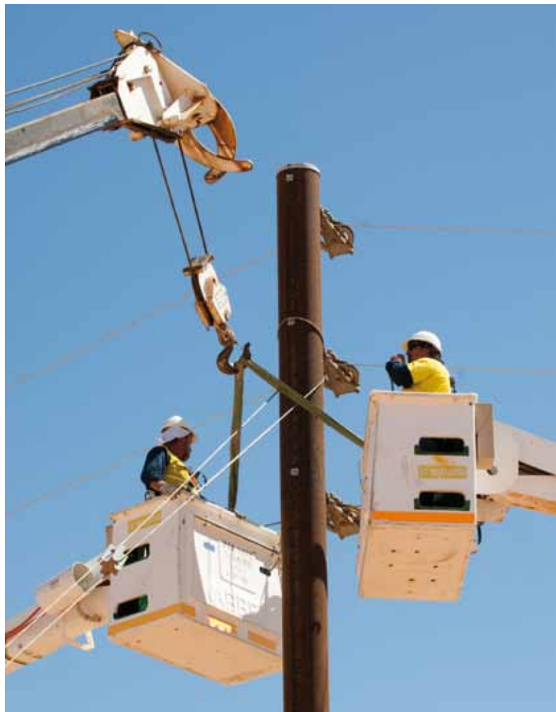
Powell Electric constructing the transmission lines to Innamincka
