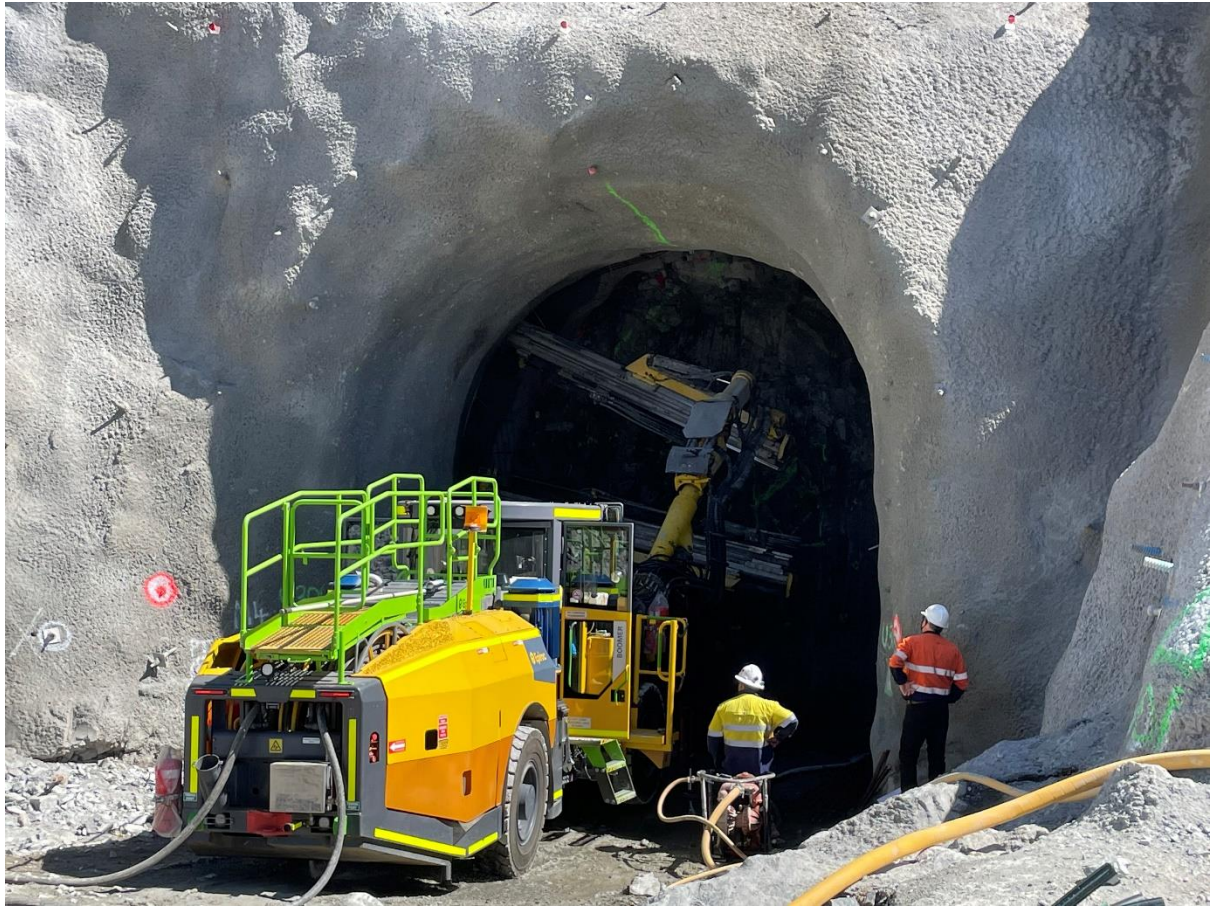
Figure 1: Tunnelling of the MAT – Drilling Jumbo installing Rock Bolts
