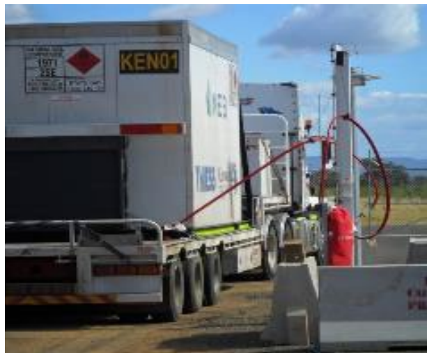
Figure 4: Loading post and filling of virtual pipeline trailers.
