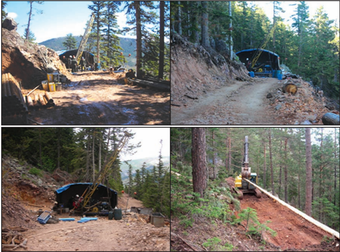
Figure 6. Selected photos of drilling and road preparation from the Sisorta project
