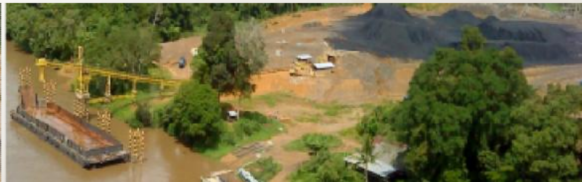
Mamahak Project – Port facility and stockpile area with conveyor and barge
