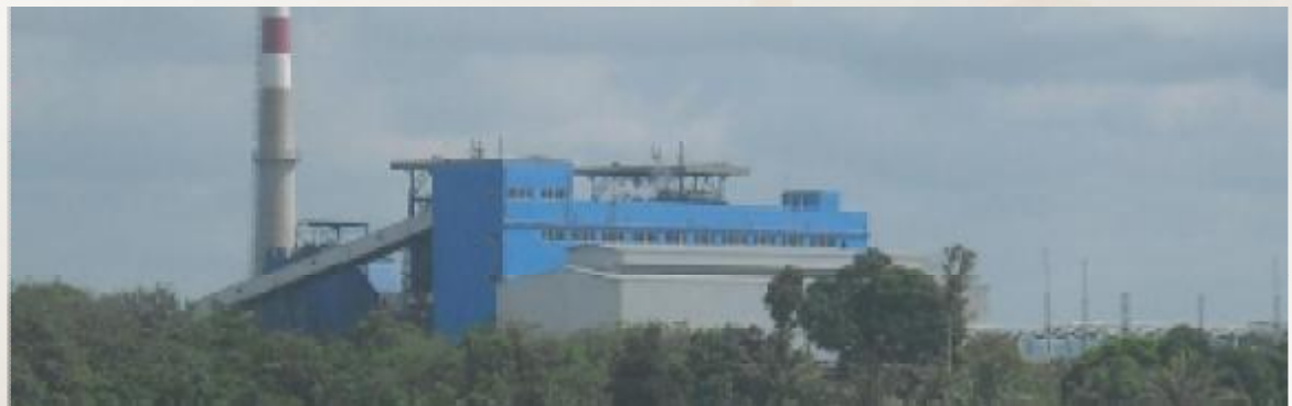
PLN power station in East Kalimantan
