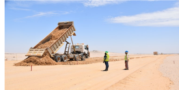
Wide haul road constructed with 100 mm gypsum running board
