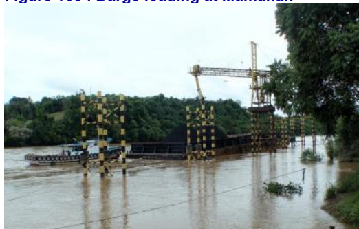
Figure 16c : Barge loading at Mamahak
