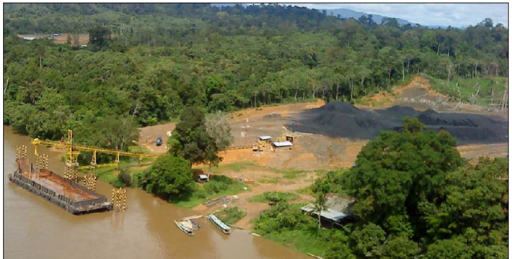
Figure 4. Barge Loading Facility at Mamahak with stockpile
