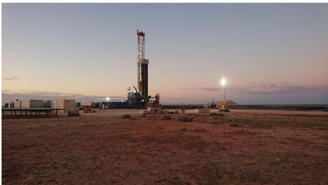
Figure 2: SLR184 rig drilling Odin-1
