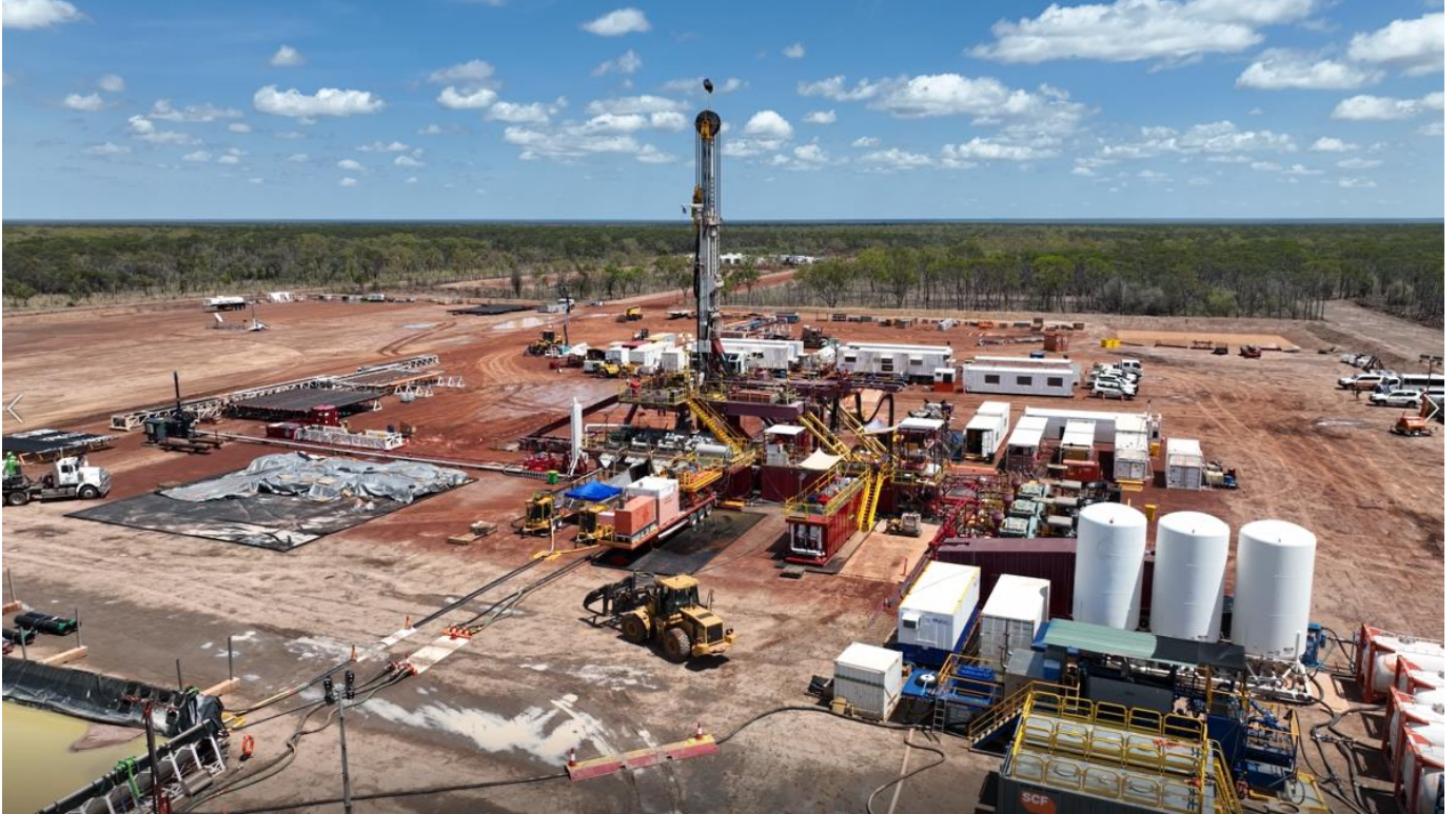
Figure 2: Drilling of Amungee 2H well on the Amungee well pad in EP 98.
