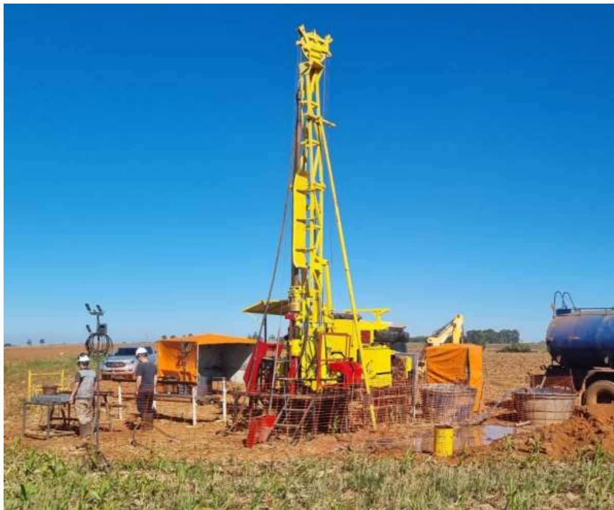
Above: Drilling at the Tiros Project
