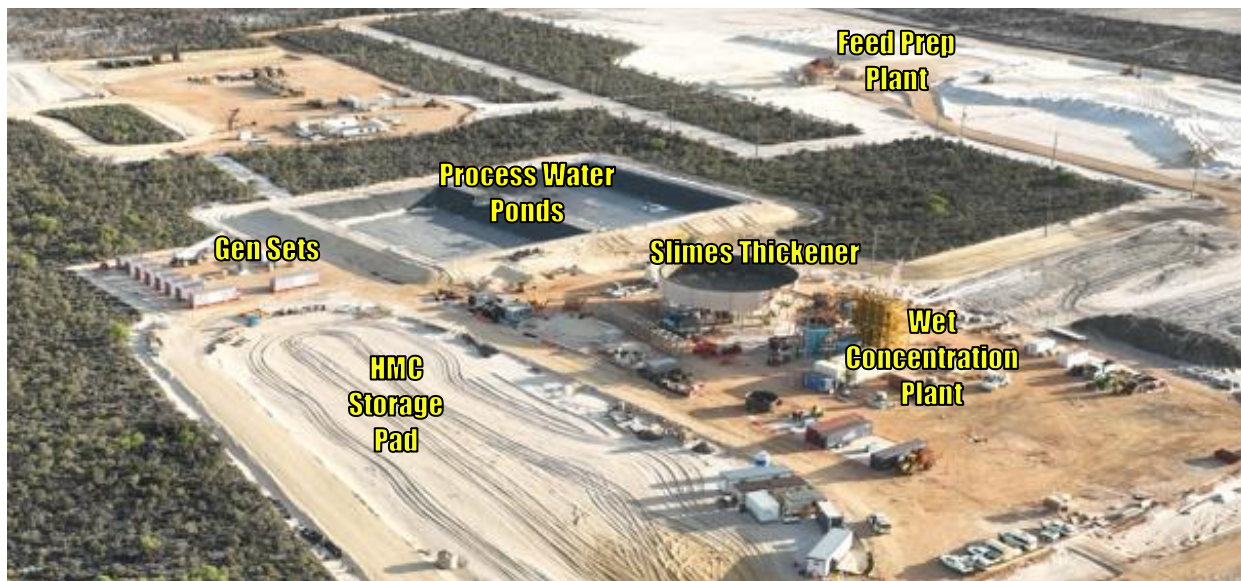
Photo 1 - Atlas Project Construction Progress - 31 December 2024
