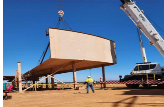
Boonanarring WCP Dismantling
