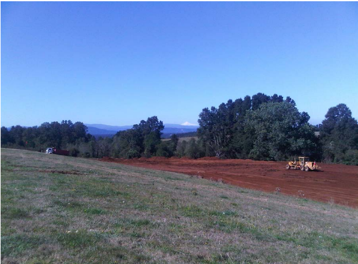
Fig 4 Earthworks for plant area underway, Mulpun
