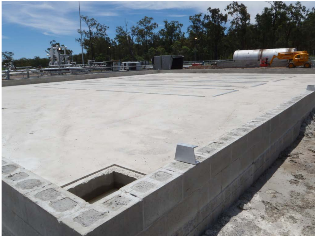
Process water facility under construction
