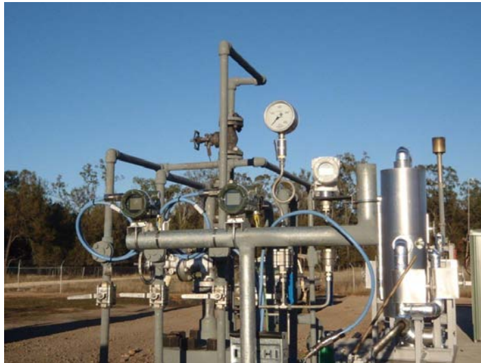
UCG Panel 2 Ignition well head
