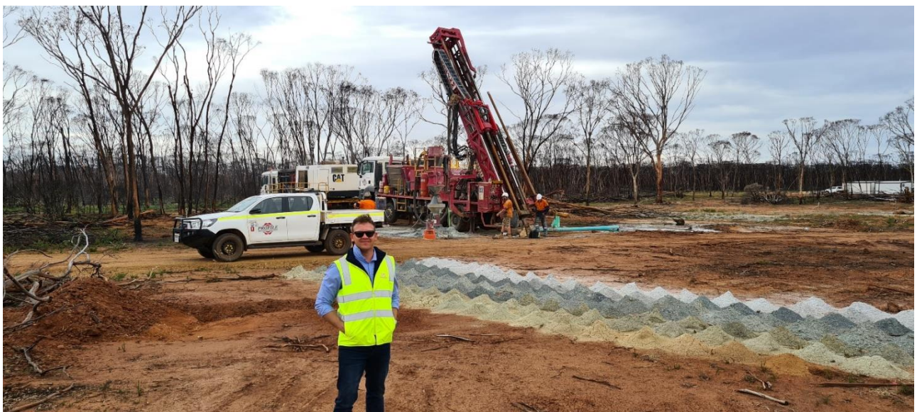
Figure 1: Drilling at Kat Gap
