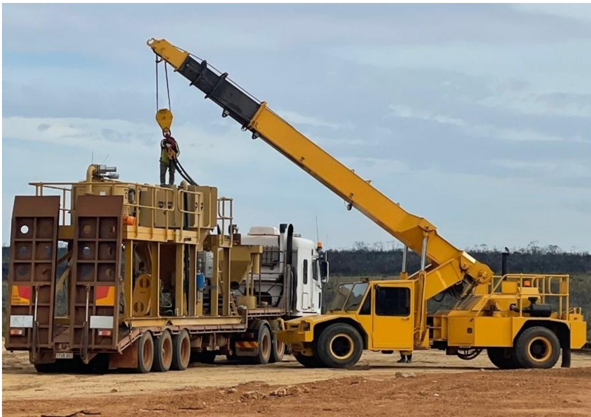
Figure 2: Loading and departure of gekko plant to Kat Gap
