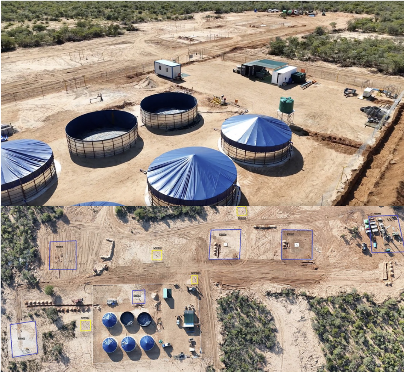
Figure 2 | Ongoing well field development at Cobre's NCP project
