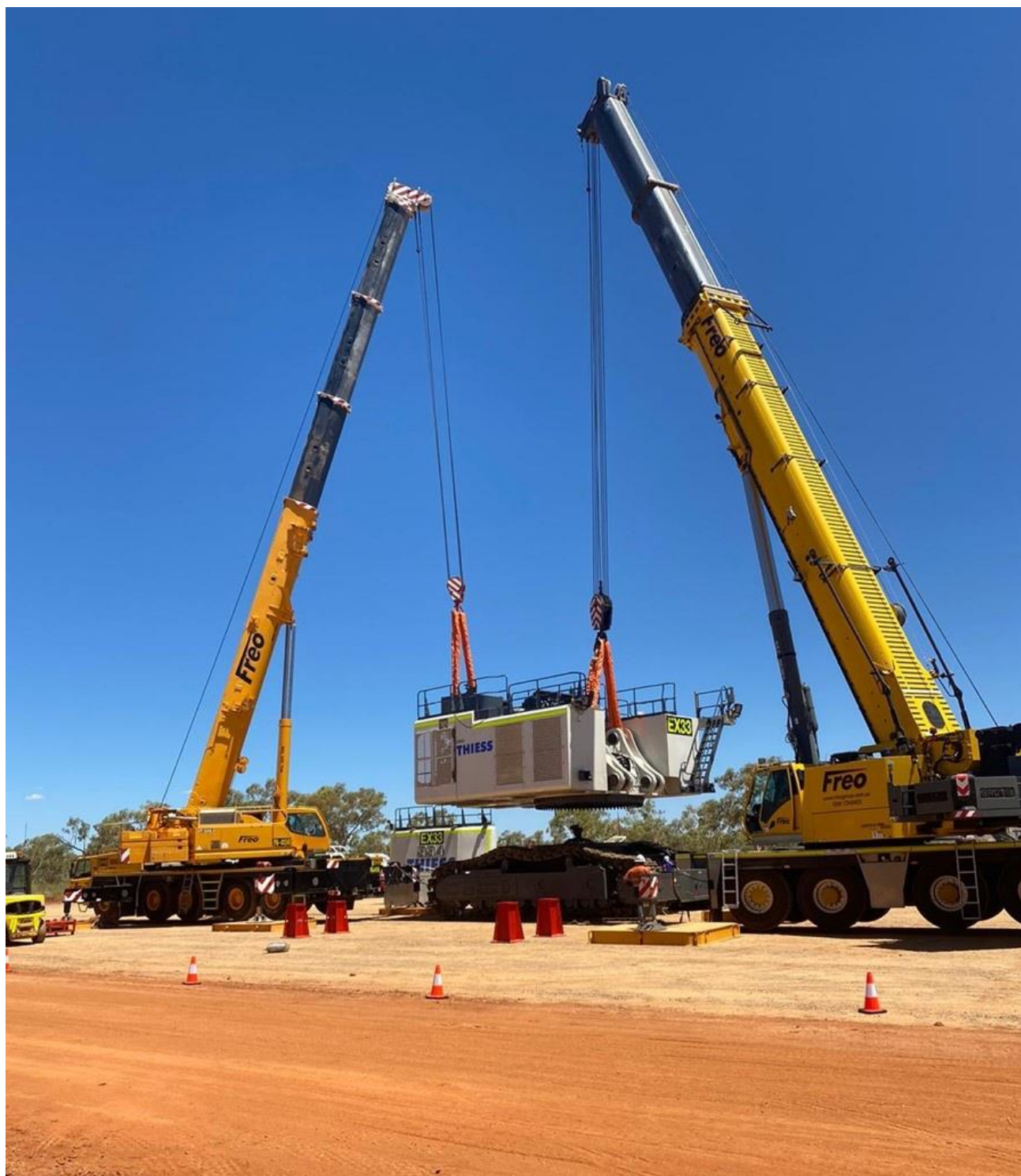
Figure 2. Assembly of the 225t Liebherr R994B at Anthill.
