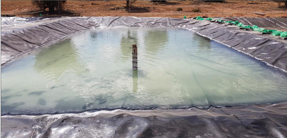
**Figure 3:** H2 one day after the transfer of concentrated brine from H1 showing immediate K salt crystallisation
