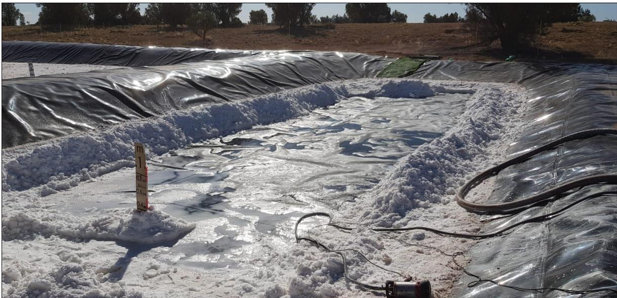
**Figure 2:** Harvest Pond 1 with stockpiled K and SO<sub>4</sub> bearing salts after brine transfer into Harvest Pond 2
