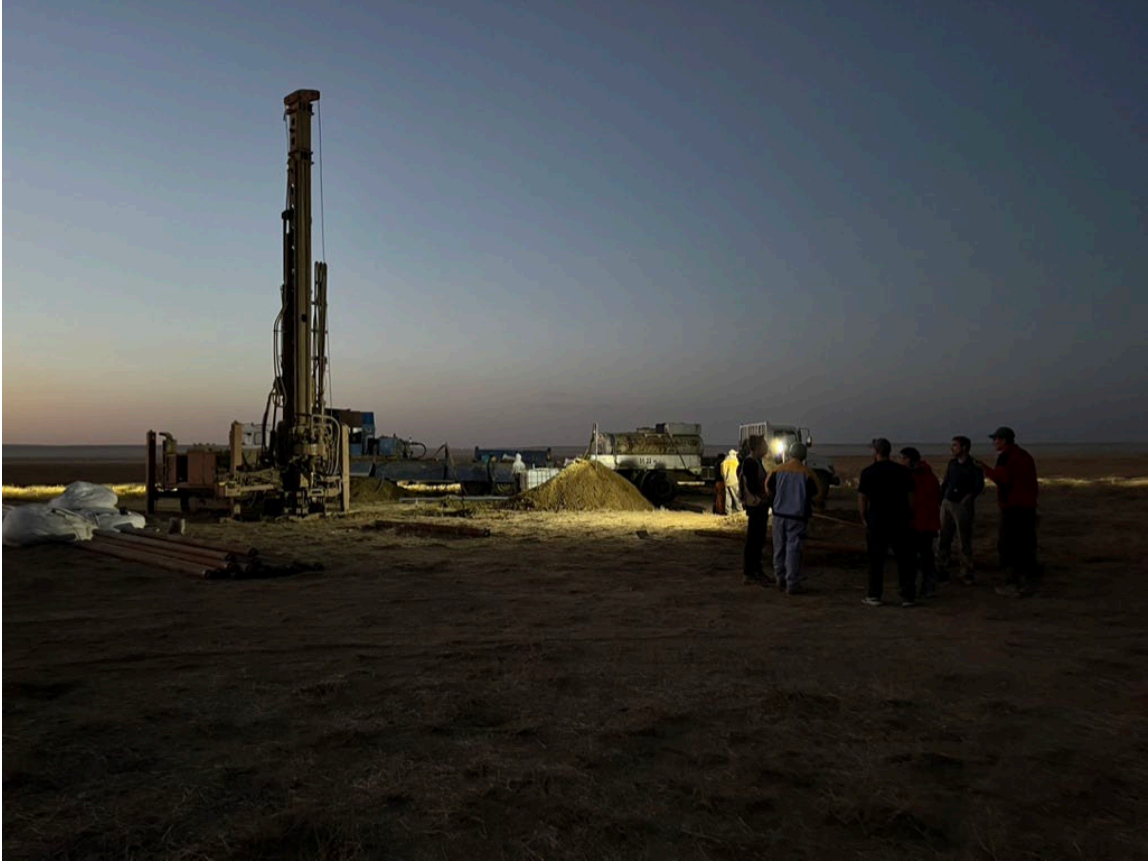
Figure 3. Waterwell rig at UNWH-01, Urgakh Naran.
