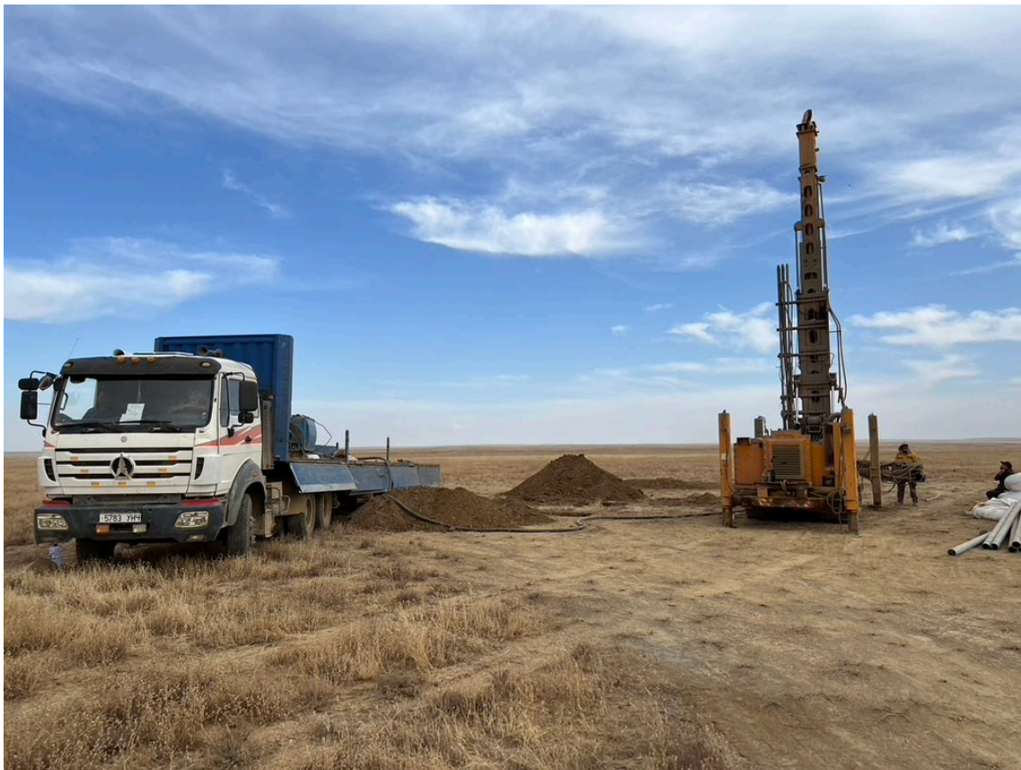
Figure 2. Waterwell rig at UNWH-01, Urgakh Naran.
