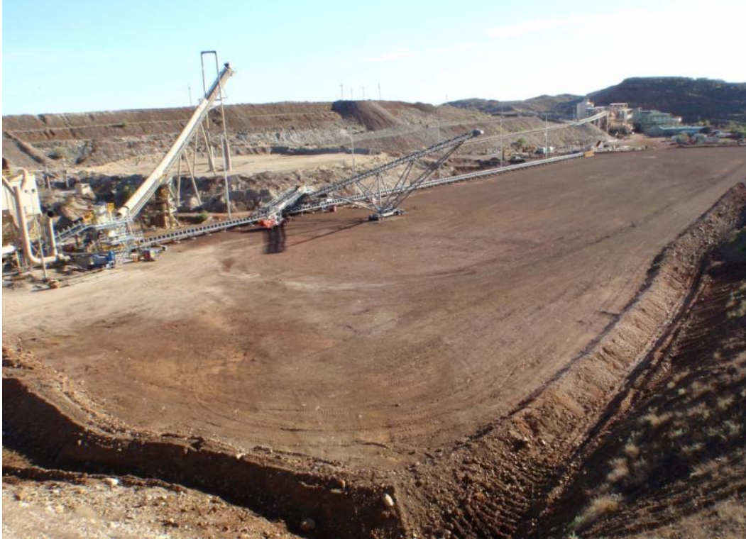
Figure 3: New Wodgina infrastructure, Stacker/Civil Works/Final Product Stockpile
