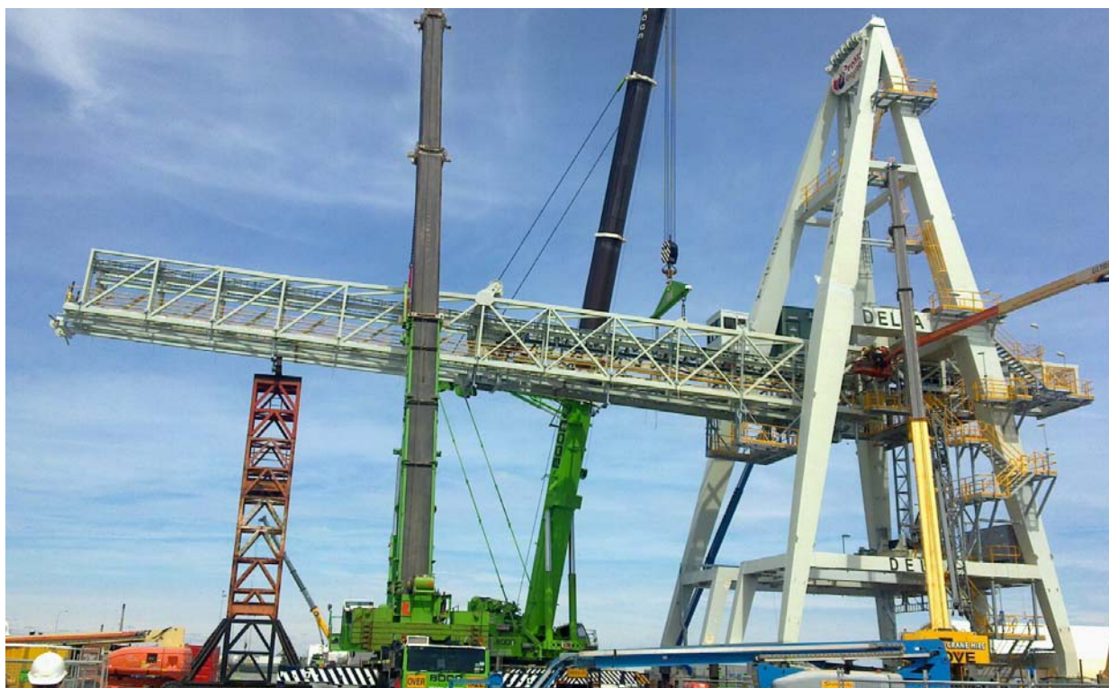
Figure 6: Utah Point Shiploader being assembled
