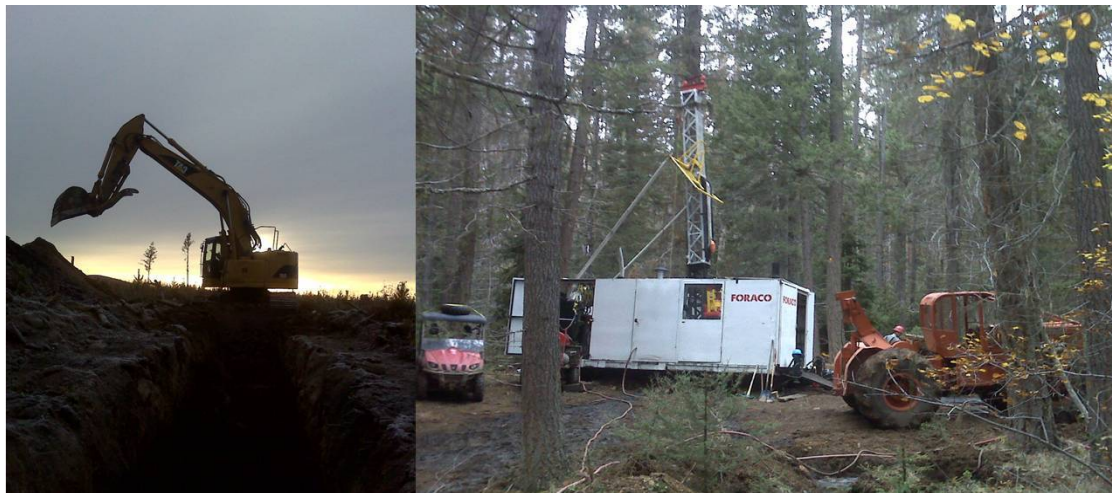
Figure 2 – Trenching and Diamond Drilling
