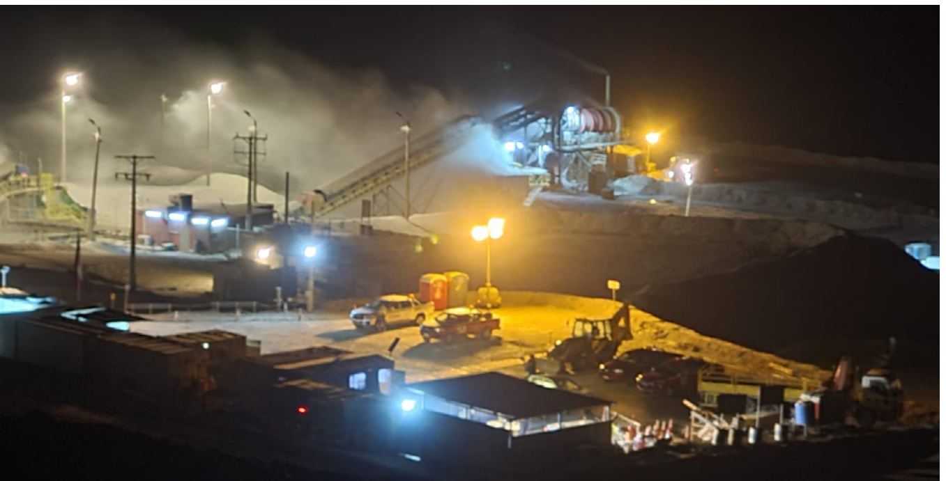
Figure 4 | Sierra Atacama crushing circuit and SX-EW processing plant
