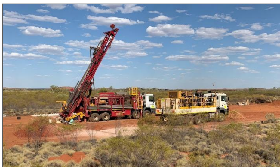
Figure 5: RC drilling rig on first hole at QXR’s Turner River lithium project - Carbonate Hill area.
