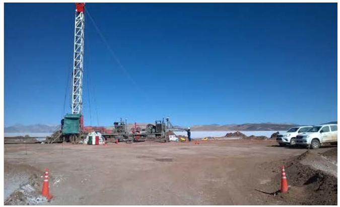
Drill Site Two Pad
