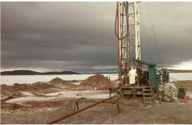
North Basin Drill site
