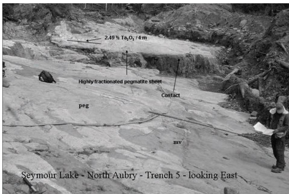
**Figure 7.** Overview of Trench 5 at North Aubry prospect showing the tantalum mineralisation.
