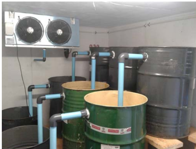
Chiller units for the evaporation / condensation process
