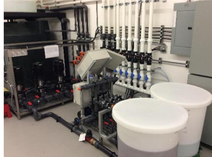
**Figure 2: Duncan Facility automated fertilizer system.**
