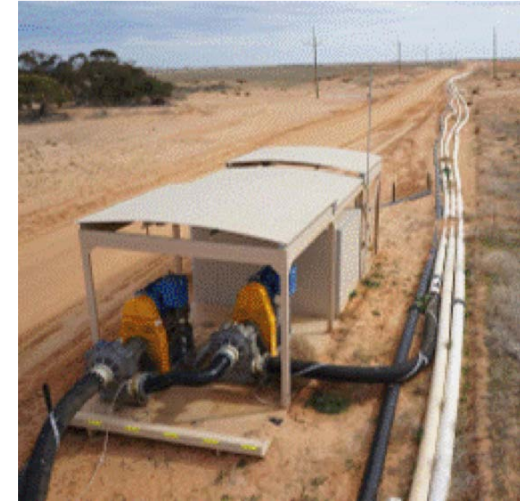
Slurry Booster Stations & pipelines
