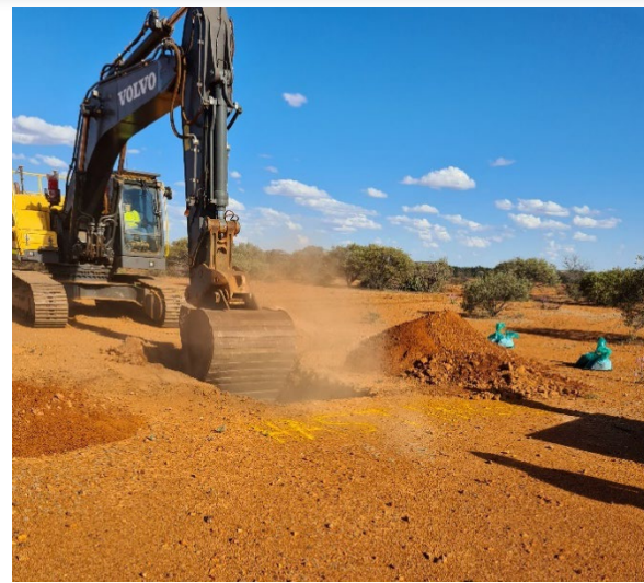
Geotechnical test pitting, August 2021
