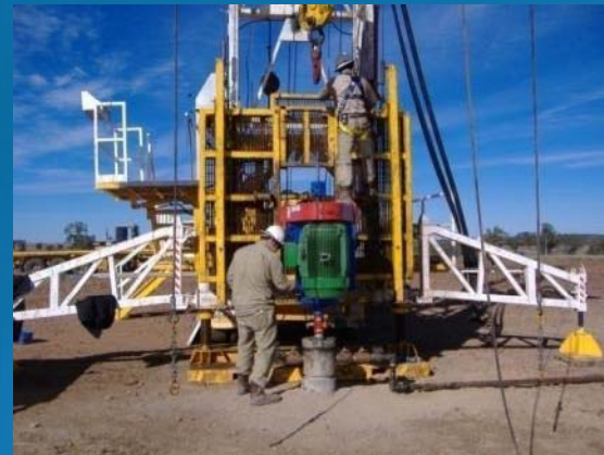
Installing an electric drive head
