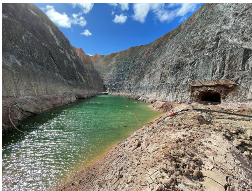
Figure 7: Dewatering progressing at East Pit now exposing another decline (on right hand side of the Figure)
