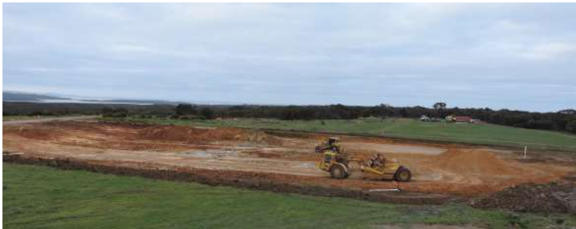
Uley Pit 2 – Pre-Strip and Overburden Removal
