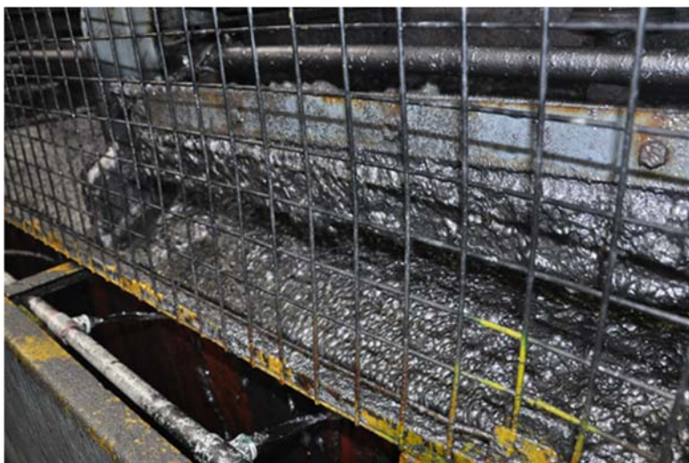
Graphite Flotation Tanks in operation
