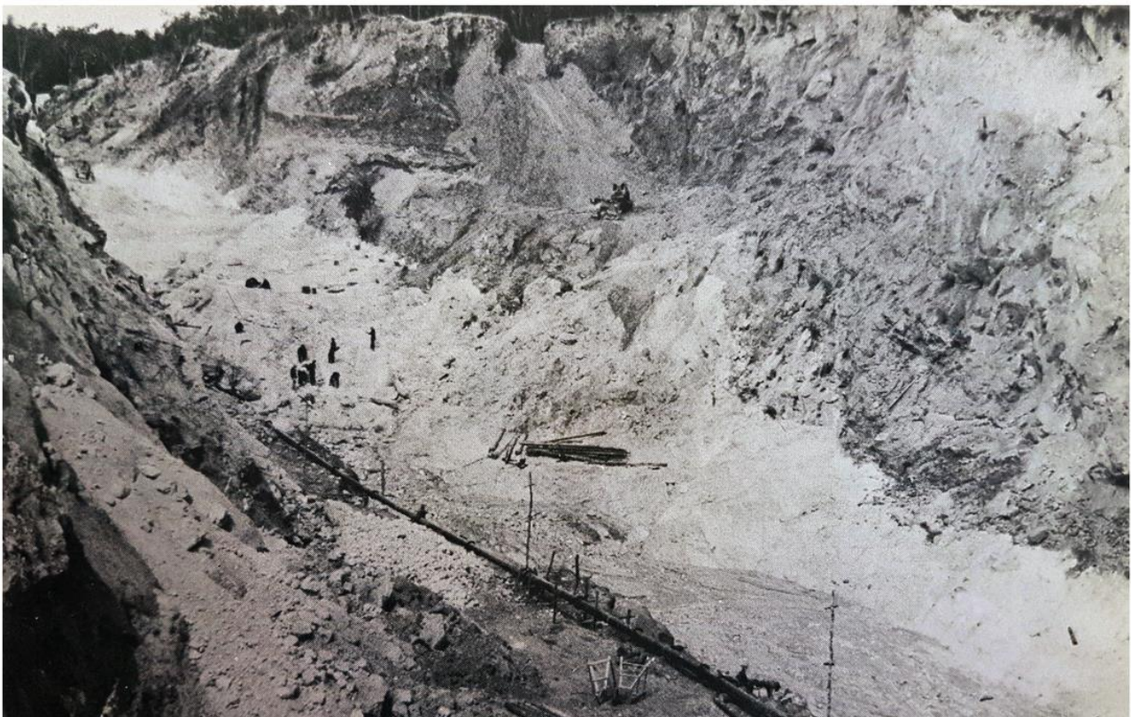
Lepidolite-pegmatite cutting mudstone of the Phuket Group, Reung Kiet Mine, 11 km south-west of Takua Thung. The light-coloured pegmatite in the lowest part of the excavation contrasts vividly with the darker coloured mudstones forming the steep slopes.
