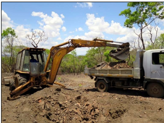
Figure 1: Excavation of bulk sample
