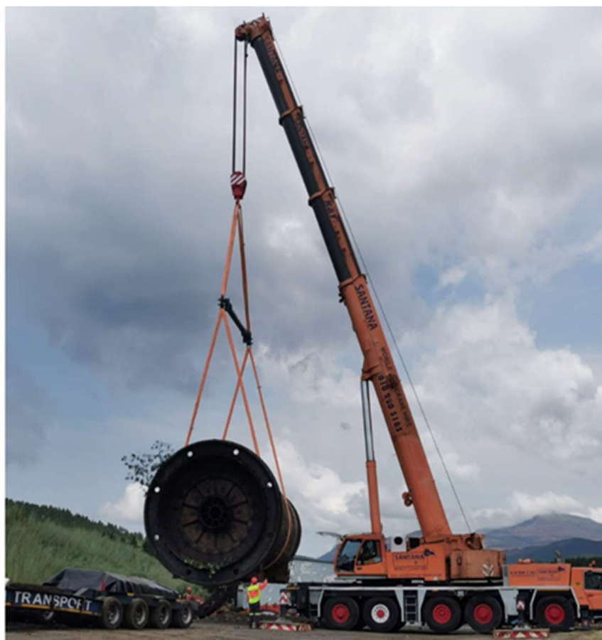
Figure 2: Ball Mill drum being offloaded upon arrival at Theta Gold's TGME CIL Plant site
