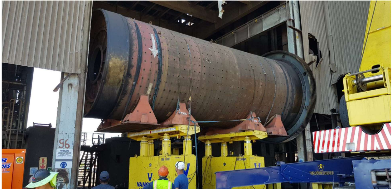
Figure 4: Mill Removal From Structure
