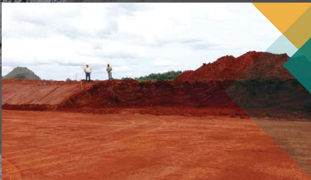
Figure 3: First excavation for ore silo foundations
