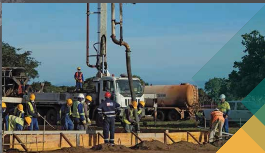
Figure 4: Pouring of floor slab for the construction of a larger accommodation camp
