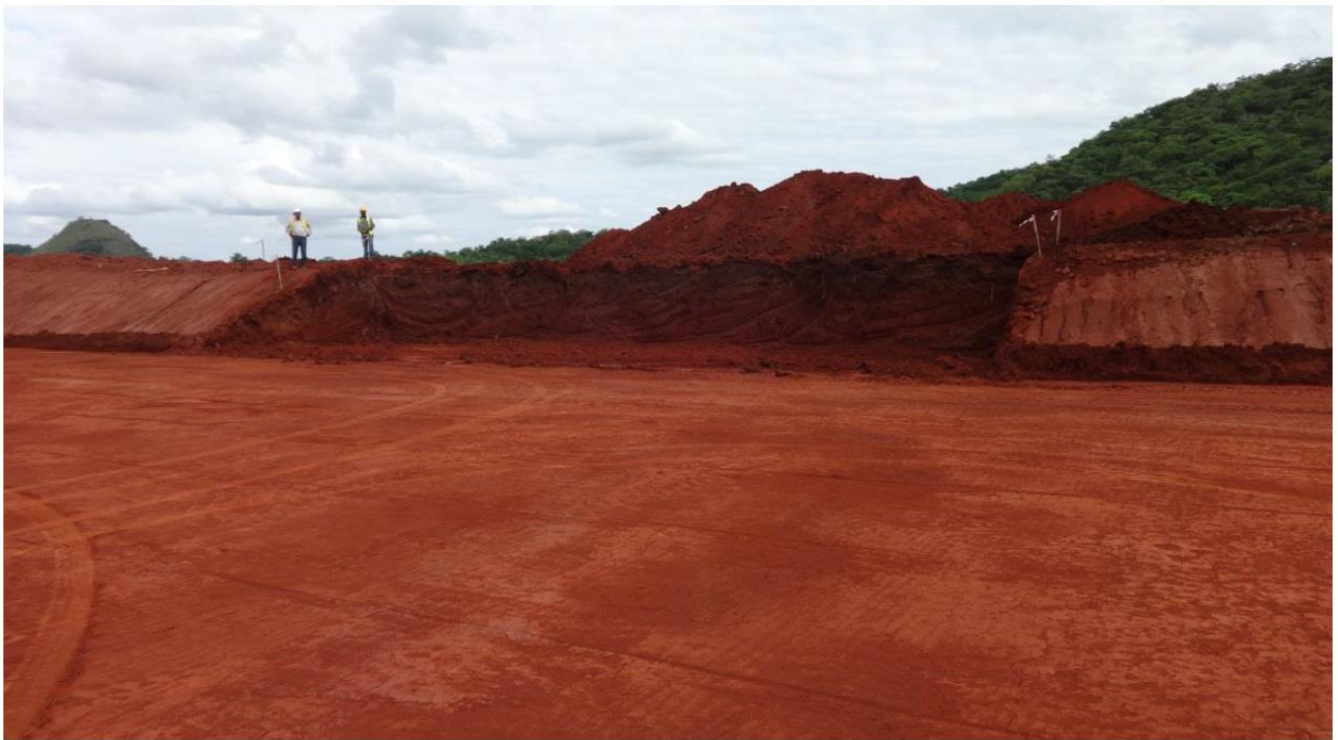
Figure 3: First excavation for ore silo foundations
