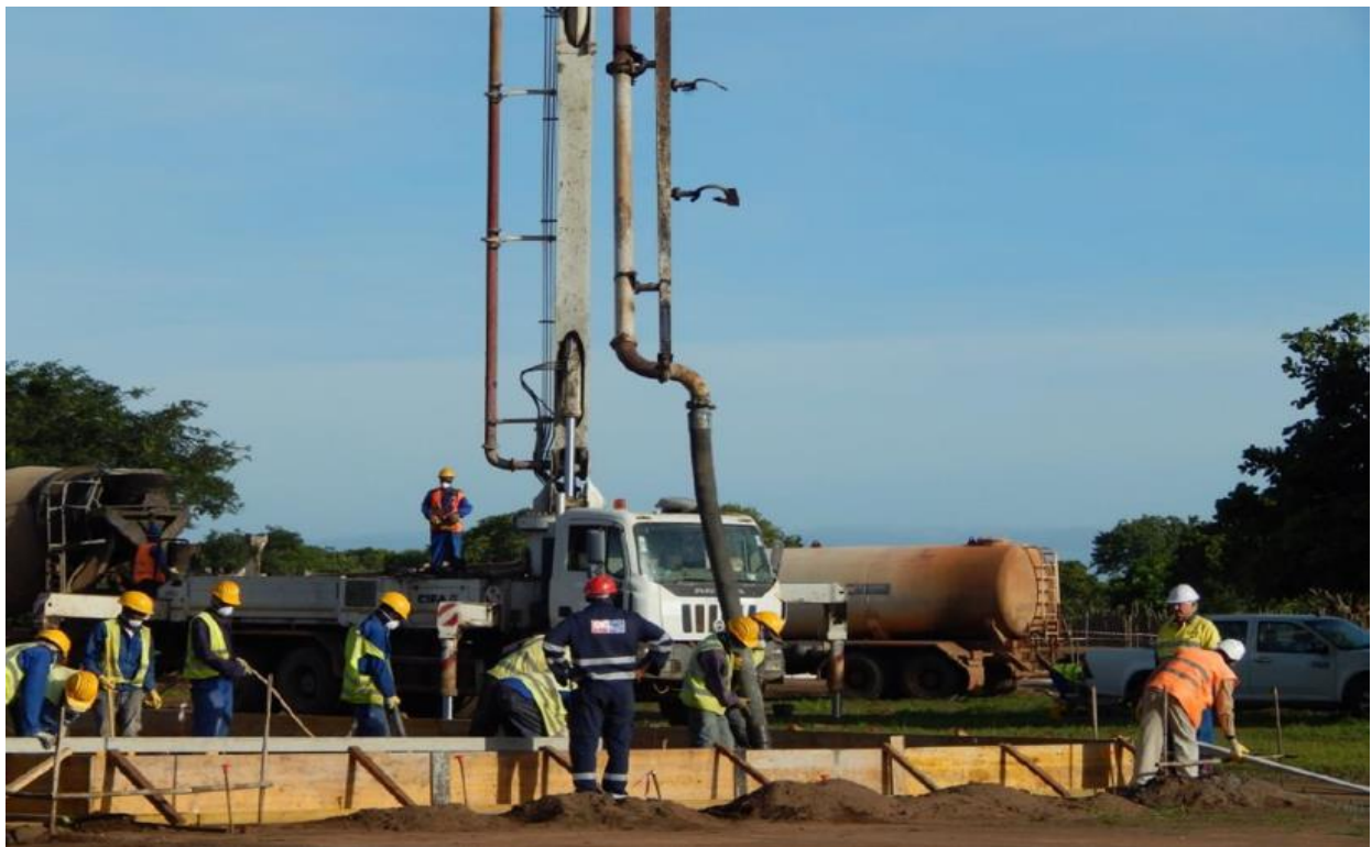
Figure 5: Pouring of floor slab for the construction of the final accommodation camp
