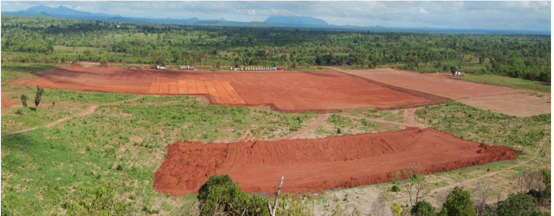
Figure 1: Cleared process plant site with completed bulk earthworks
