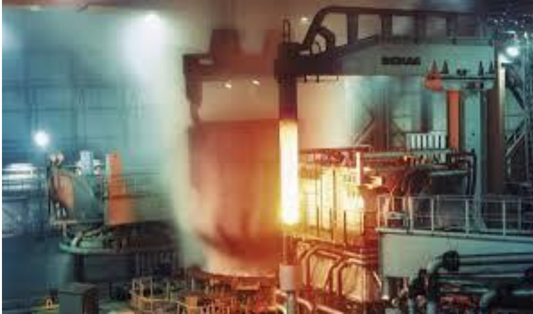
Figure 1: Electric arc furnace
