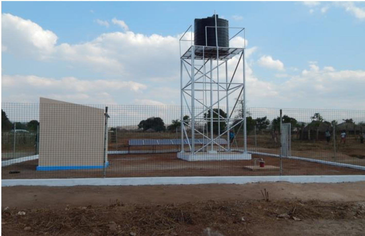
Community water facility installed at a local village
