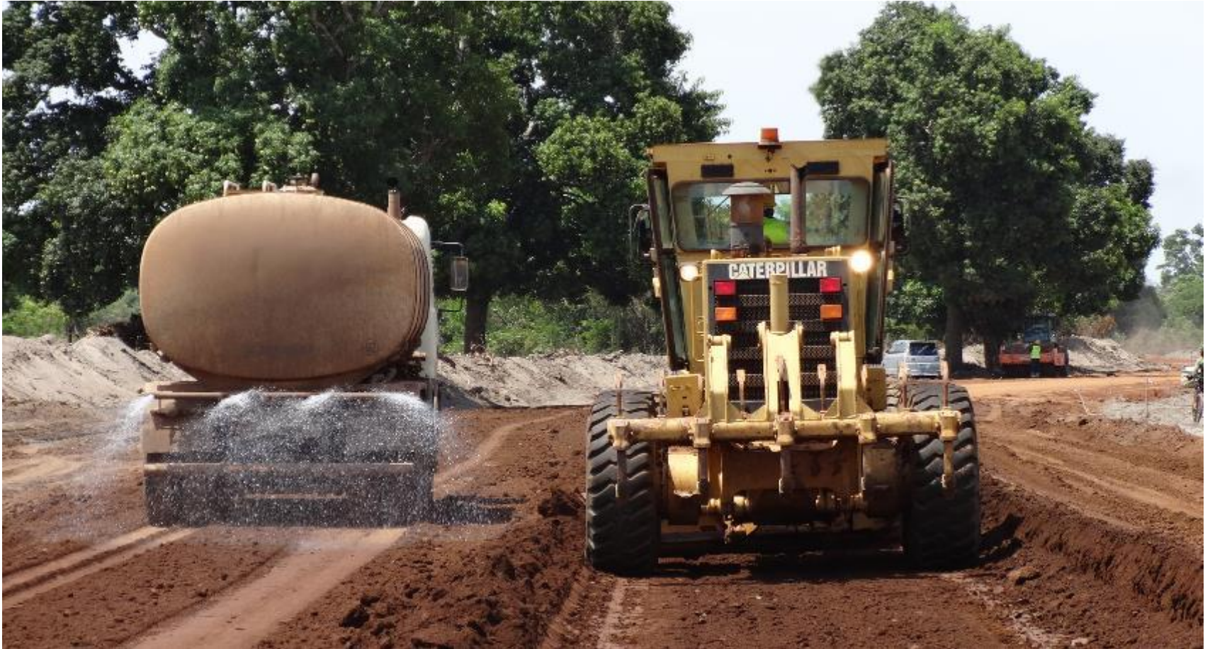
Process plant access road being laid
