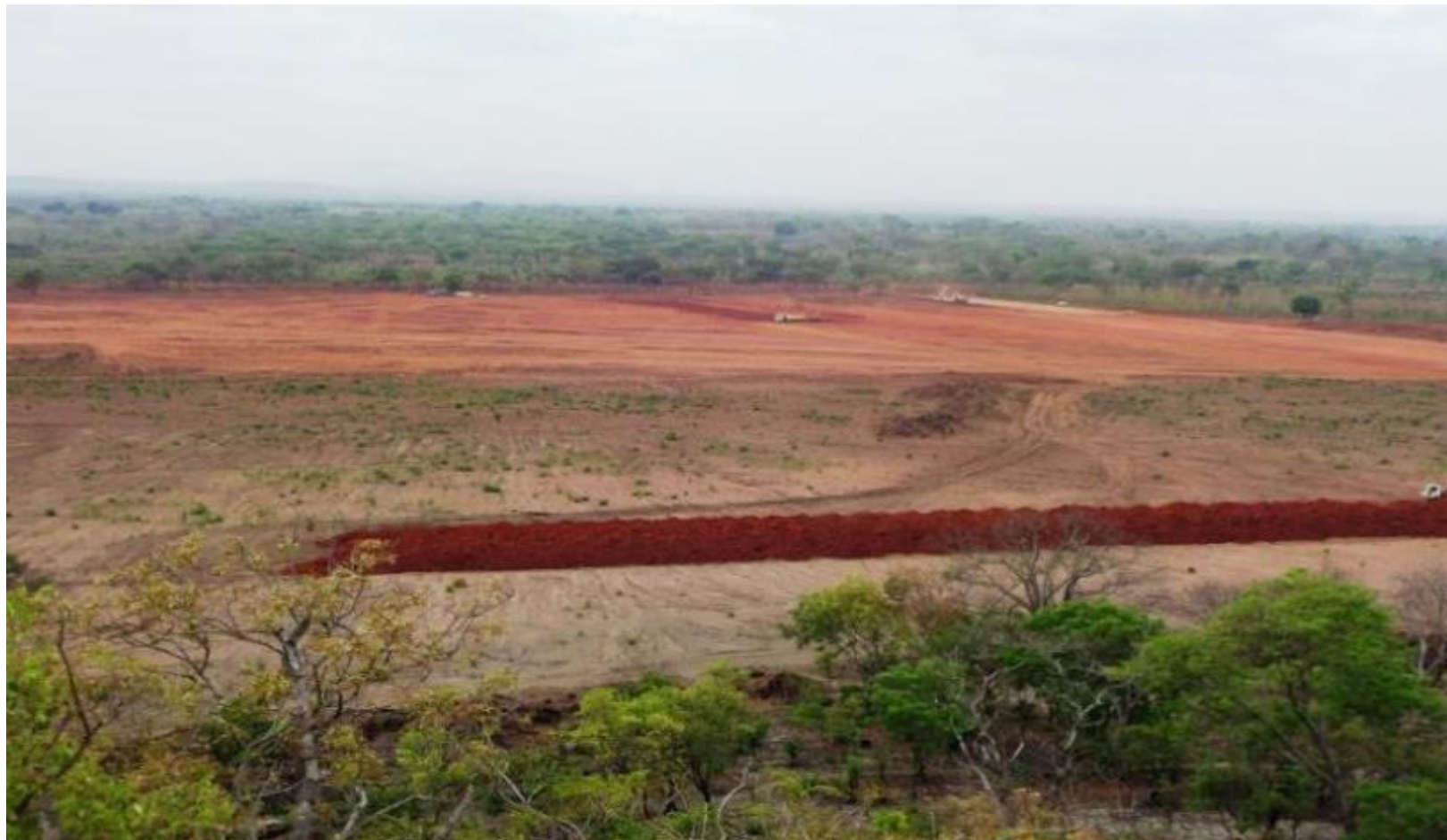
Bulk earthworks at the Balama processing plant site
