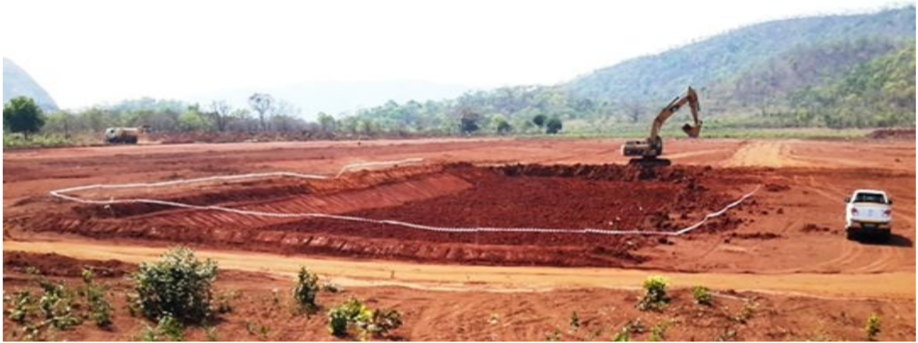
Figure 1: Excavated area for the Balama processing plant
