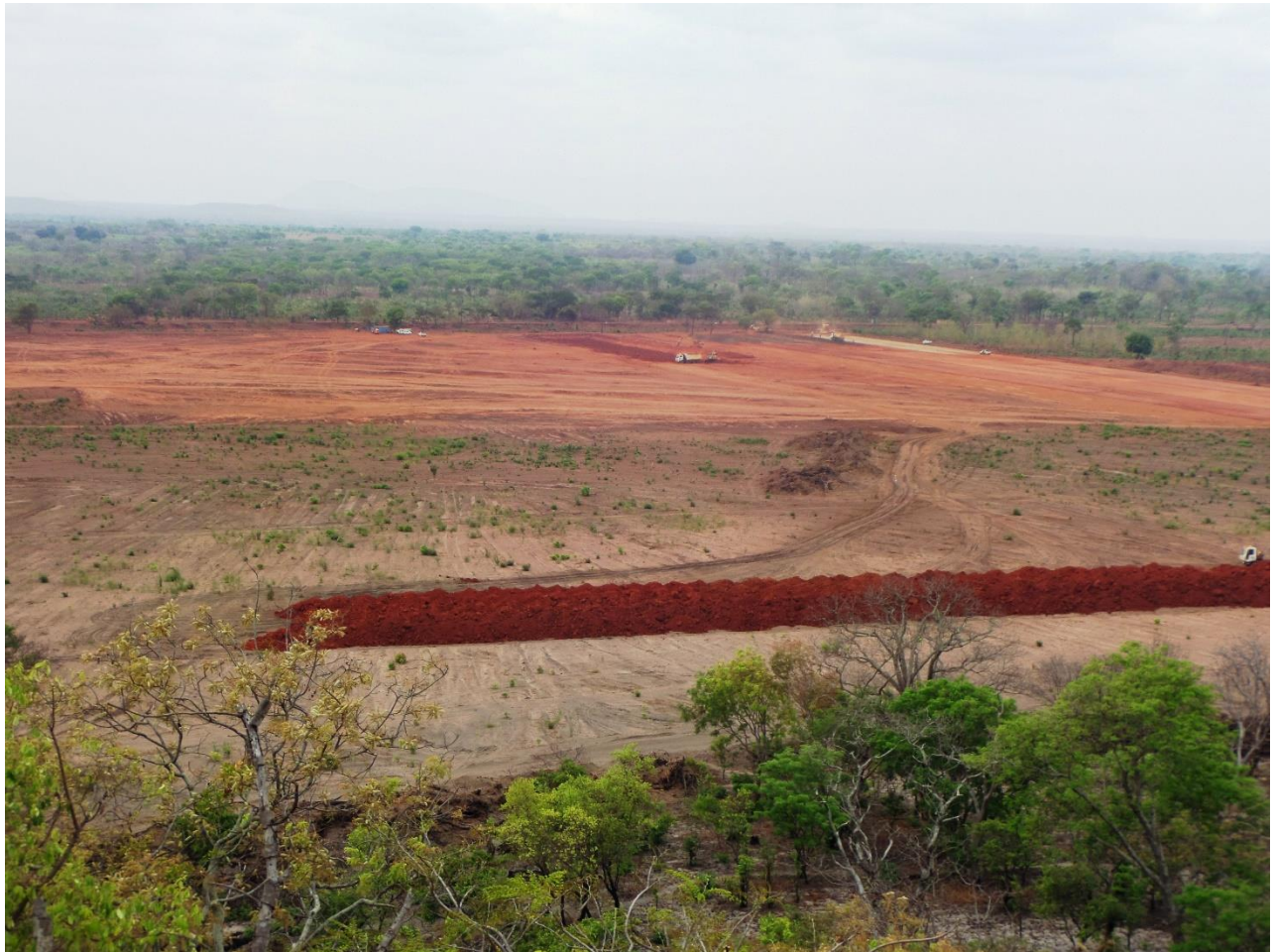
Figure 2: Bulk earthworks at the Balama processing plant site
