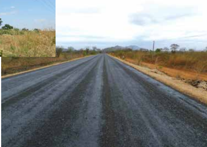
Figure 6 – Bitumen road to the Balama Project
