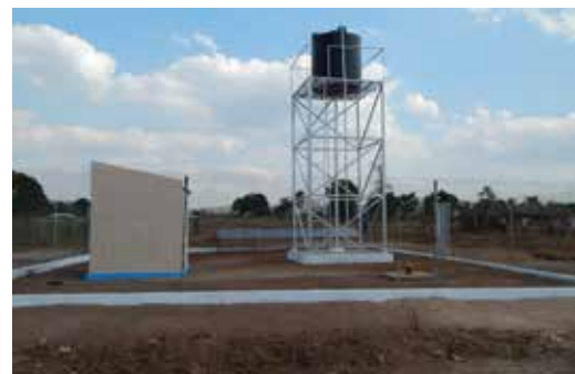
Figure 12 – Community water facility installed at a local village
