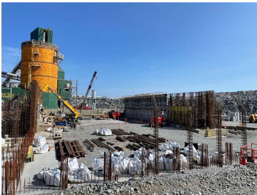
Figure 1 North American Lithium – Crushed Ore Dome side wall construction
