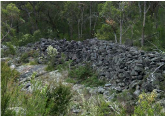
Stone wall several metres high with individual blasted blocks up to five tonnes that were hauled in 1863 by two-man winch team from the basement of Kentucky Creek. A very rare feature in a 19 th century alluvial goldfield; the effort and resources expended is a testimony to richness of the gold along this portion of Kentucky Creek.
